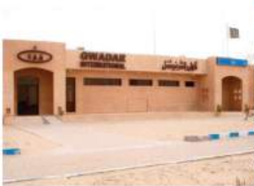
Existing Gwadar Airport
