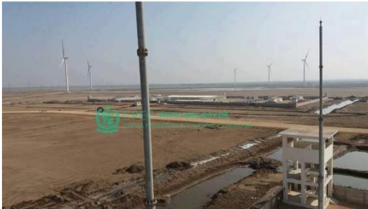
Hydro China Dawood 50MW Wind Farm (Ghara, Thatta)(COMPLETED)
