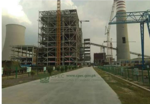
Sahiwal 2x660MW Coal-Fired Power Plant, Punjab (COMPLETED)
